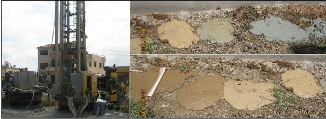
Figure 3: Drill chipping samples collected during drilling
